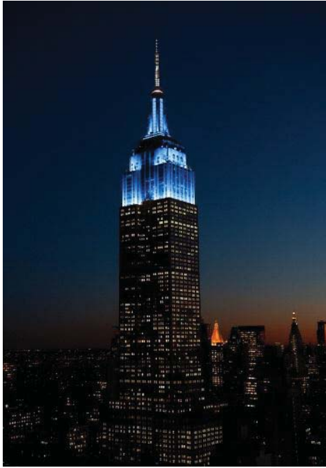
Fig. 4 Empire State Building
