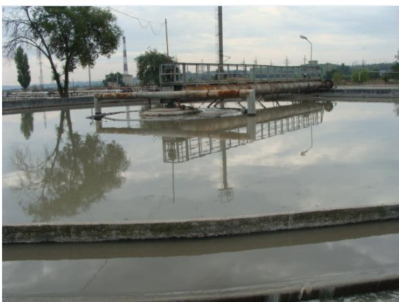
Fig. 1.3. Decantor radial primar
