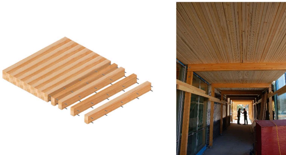
Figura 3. Nail-Laminated Timber (NLT) [2]
