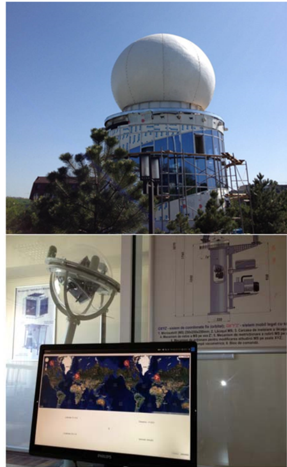
Figure 2. CNTS ground station.
