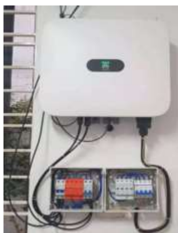
Fig. 4.11. Invertor On-Grid Huawei solar SUN2000-3KTL-M1 [114]
