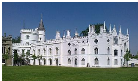
Figure 1: Strawberry Hill House in 2012 after restoration
