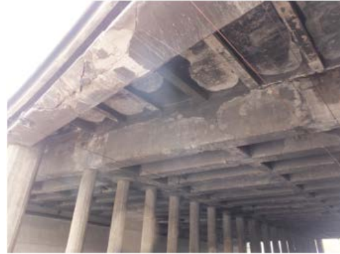
Figure 7. The marginal girder.
