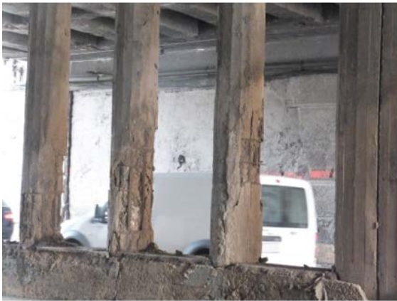
Figure 4. The Constanța Bridge pier before rehabilitation works.
