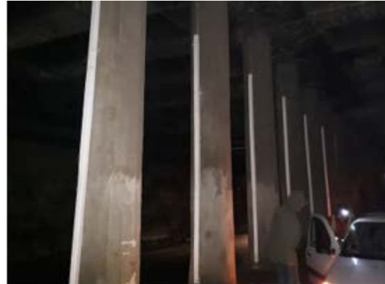
Figure 18. Installation of optical fiber at the pile column.
