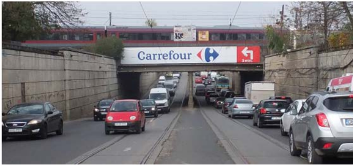
Figure 1. The Constanța Bridge.
