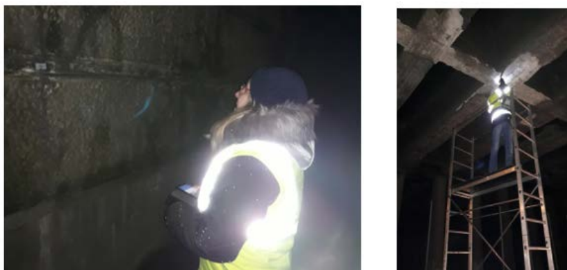
Figure 16. Data capture for structural reinforcement.
