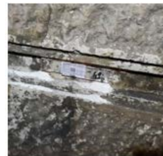
Figure 10. Glass marker for monitoring crack evolution.
