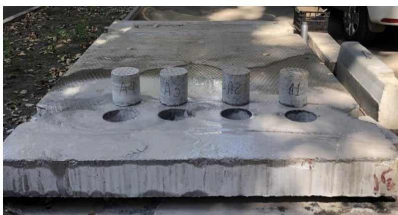
Figure 7. Drilled cores of the slab
