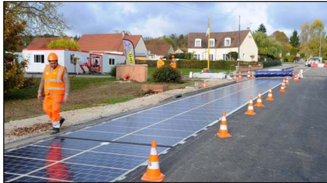
Figure 3. Wattway panells pavement.
