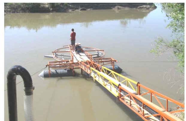
Figure 23. Micro hydropower station MHCF D4x1,5E installed on river Prut.
